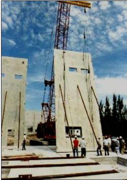
Tilt-up Concrete Walls
