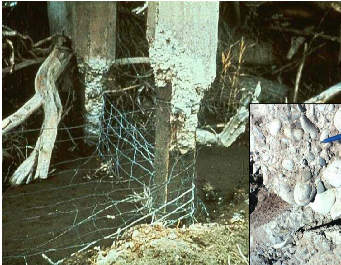
Bridge columns in North Dakota in sulfate soils
