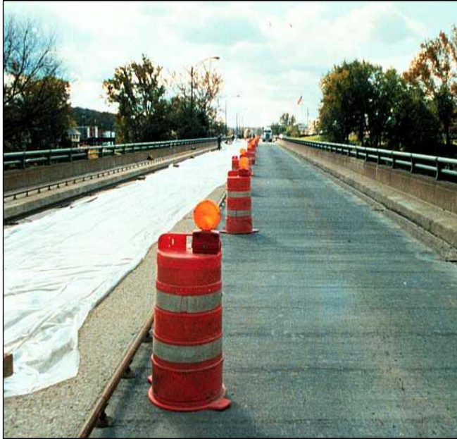
Bridge Deck Overlay
