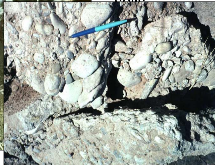
Bridge columns in North Dakota in sulfate soils
