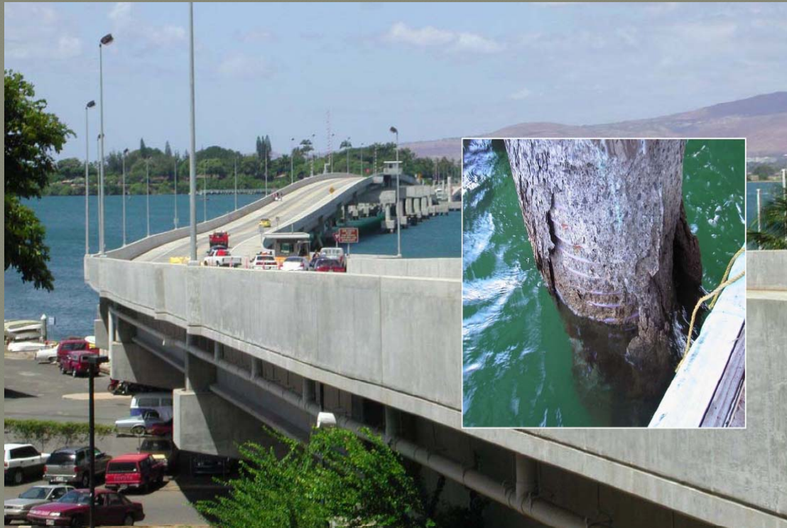
Admiral Clarye Bridge, Pearl Harbor, HI
